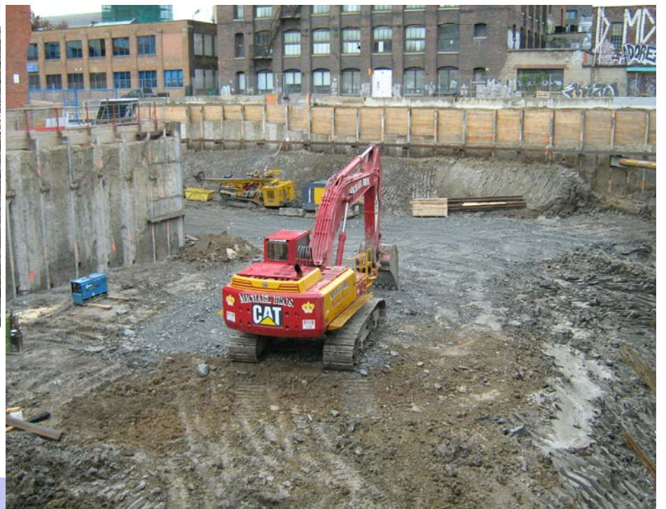
Impacted soil at a condominium redevelopment site, Toronto, Ontario
